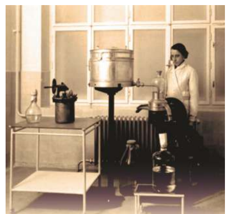
Centrifugation of pig blood in an ALFA Laval flow centrifuge (1936)
